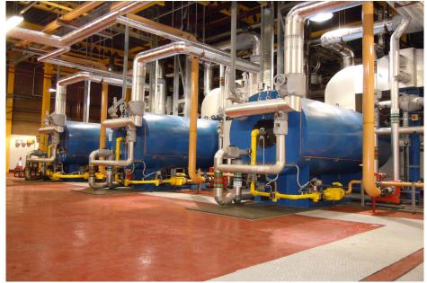
is confined in a restricted space and is heated by burning a fuel source. The energy of combustion is transferred from the flame to the water by radiation and conduction, heating the water and ultimately raising steam. However, the means of heating the water to the point of 'dry' steam are markedly different and have resulted in one being the modern day champion.
